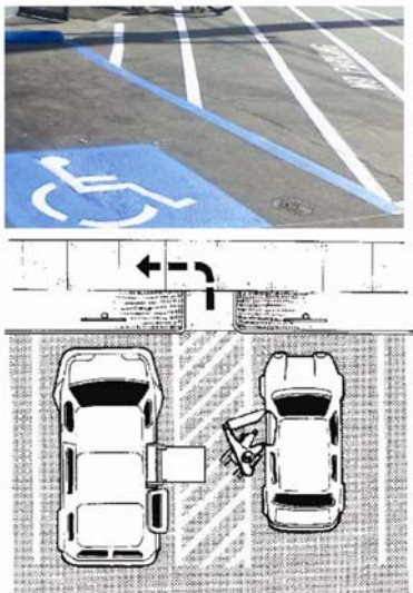
Sample Access Aisle with Contrasting Lines
